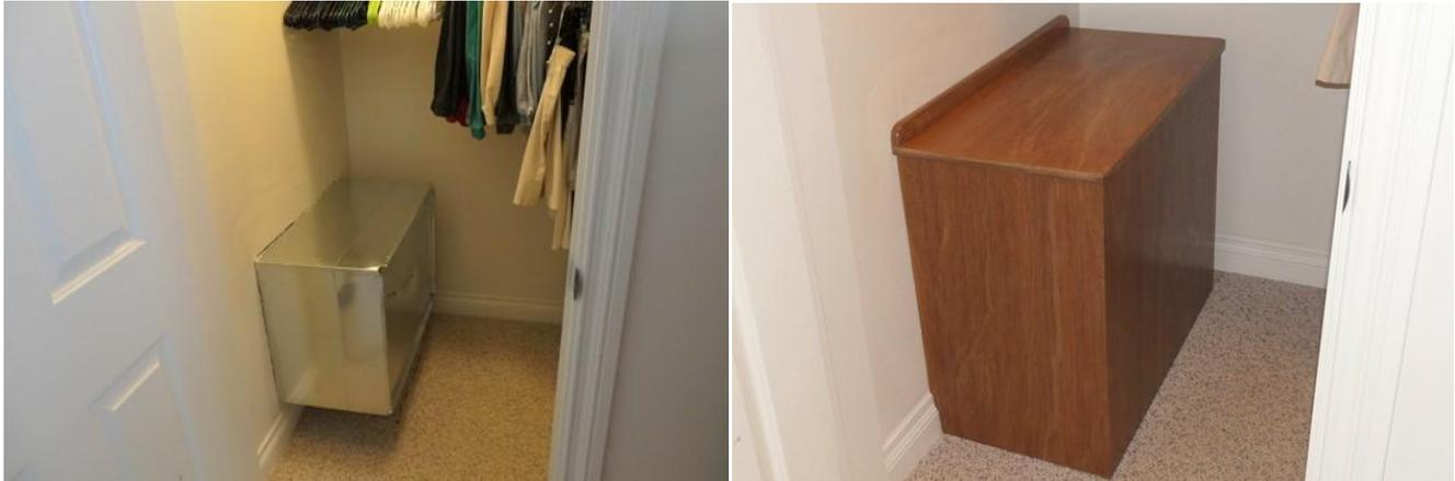
I built a cover for a sheet metal plenum in one of our closets. The plenum was needed for a new furnace that replaced our old furnace, which had failed in January. The new furnace did provide improved zoning plus reduced noise level. However, a second return air duct was required, which meant cutting a hole in the wall between the closet and hall plus a hole in the floor of the closet for a custom made plenum.
